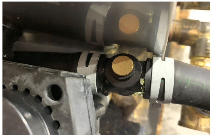
Fig. 24b Valve brass bleed screw
